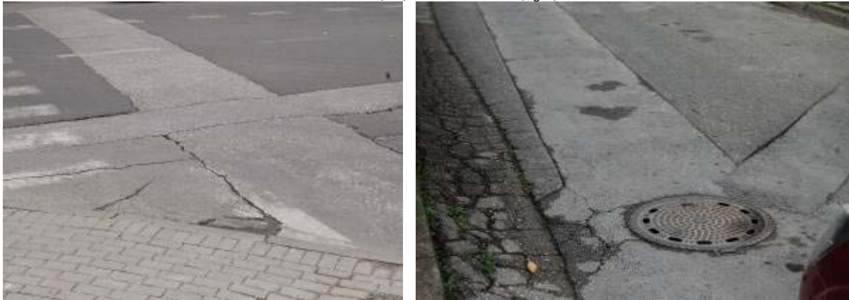
Picture 1.4. Present condition of the streets “Prashka” (left) and “Strushka” (right)
