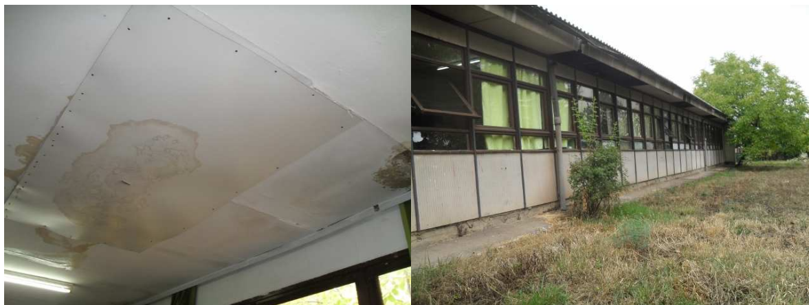
Figure 4. Elementary school Grigor Prlicev; current situation
